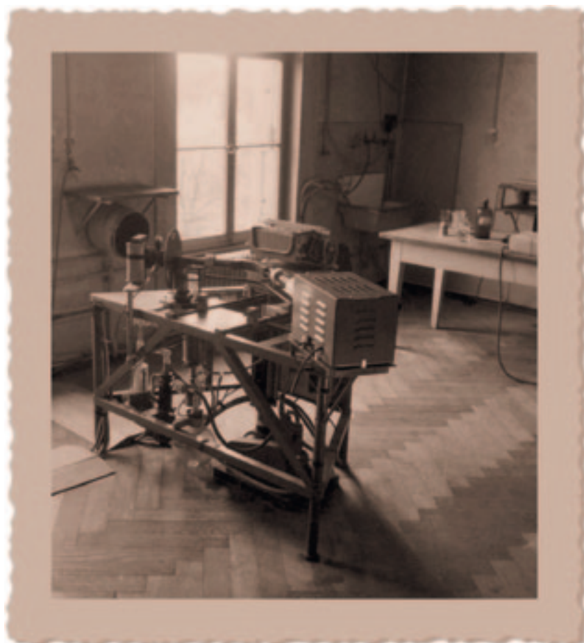
Fig. 5: The mass spectrometer Susanna 2 installed at the Physikalisches Institut in Bern, around 1954.
