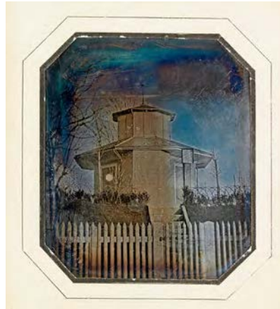
Fig. 12: Daguerrotype of the observatory “Uraniae” made by F. A. Gerber in autumn/winter 1845. The view is from the west side, so that the meridian slit is not visible. The cupola was used as planetarium. (Credit: Library of the ETHZ, KGS-454-0)
