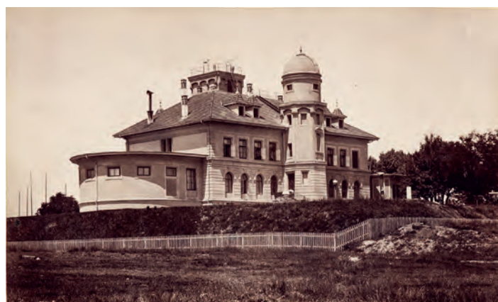
Fig. 23: Photograph of the new Observatory or Physics Institute of the University of Bern taken before 1880, showing the large lecture room on the left hand side of the two-story main building, the meridian hall at its right hand side, and the two towers, the squared one used for meteorological/geophysical observations and the round one carrying the dome used for astronomical observations. (Credit: BBB, FPa.10 Nr. 46)
